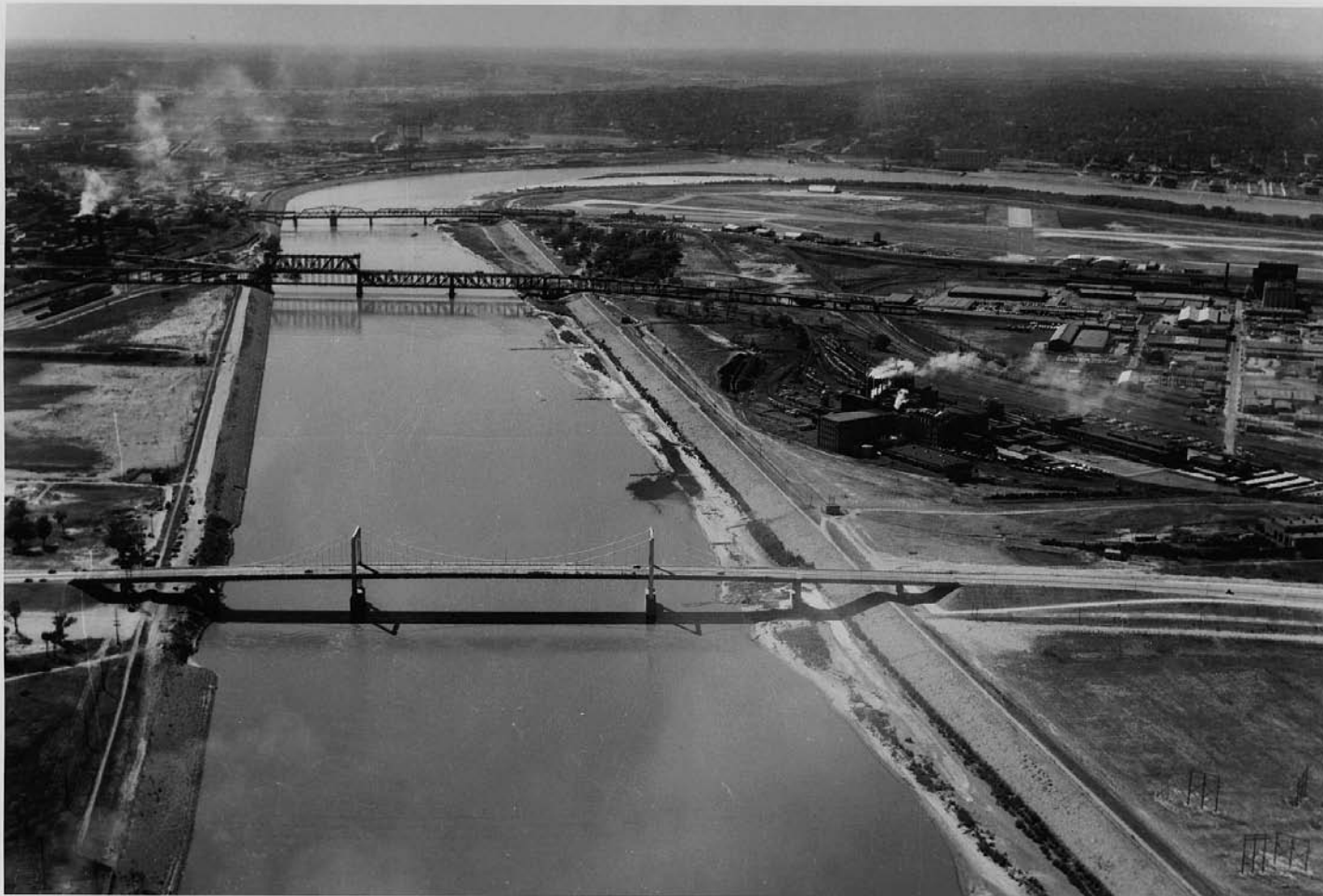
KANSAS CITY DISTRICT AERIAL VIEW WEST (UPSTREAM) FROM APPROXIMATE RIVER MILE 376, SHOWING PORTION OF RIVER FROM KANSAS CITY REACH TO KANSAS RIVER BEND. LEVEE AND BANK PROTECTION ALONG LEFT BANK IN NORTH KANSAS CITY UNIT, LEVEE AND BANK PROTECTION ON RIGHT BANK IN EAST BOTTOMS UNIT. BRIDGES FROM BOTTOM UP ARE: NEW PASEO BRIDGE; (A.S.B.) HIGHWAY & RAILWAY BRIDGE AND E.B. & Q. R.R. (HANNIBAL) RAILWAY AND HIGHWAY BRIDGE. CONFLUENCE OF KANSAS AND MISSOURI RIVERS IN CENTER BACKGROUND. 23 SEPTEMBER 1954
